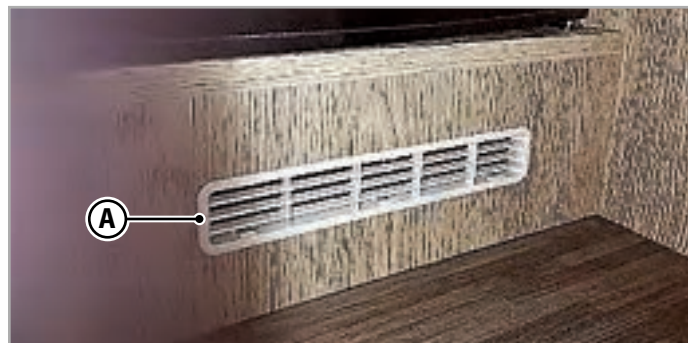
Fig.6.1 - Permanent ventilation openings
